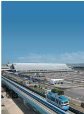
Asia's next hub: Taiwan Taoyuan International Airport
